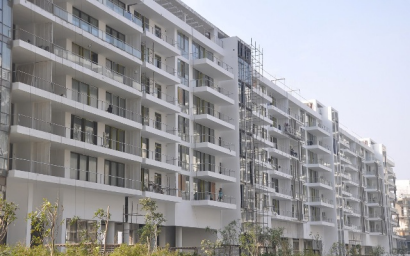
External Façade & Painting work is nearing completion
